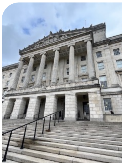
Arriving at Stormont, home of the Northern Ireland Assembly
